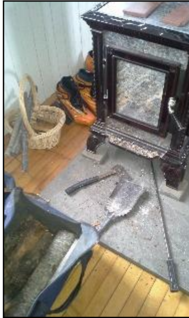
6. Floor - combustible clearance inadequate
