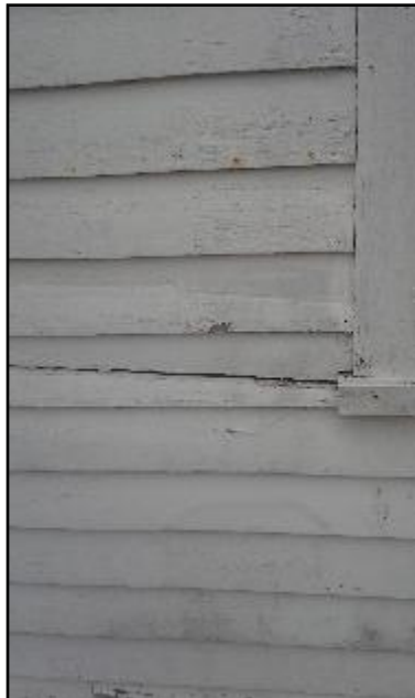
3. Cracked, split or broken
